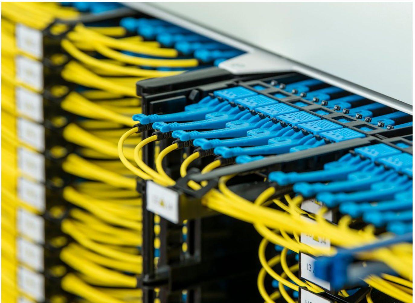
IANOS fiber management system featuring front access connectivity.
