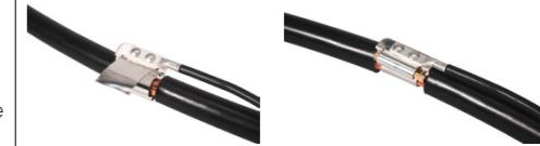
Butyl mastic is placed around the clamp and acts as a filler. The vinyl electrical tape is wrapped around the hole ground strap to make it waterproof.
