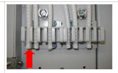
Mount the conduits with the Miniflex OFTP zipper on the loose tube.
